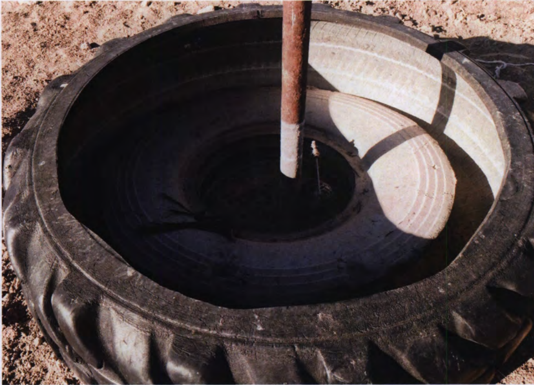
Image 16: Tire water “trough” with water marks and float valve. Cement failed to hold water. Note dead roadrunner and dead animal caught on float valve. Photo taken on July 13, 2015. Compare to Image 5. Photographed July 13, 2015.
