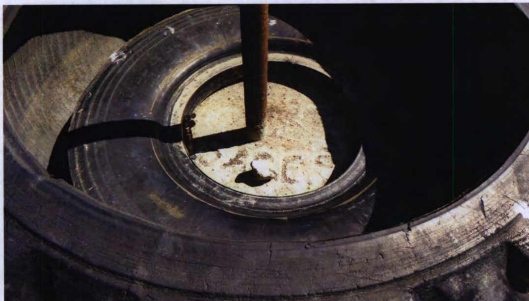
Image 5: Cemented base of the "tire water trough." Photographed May 10, 2015.
