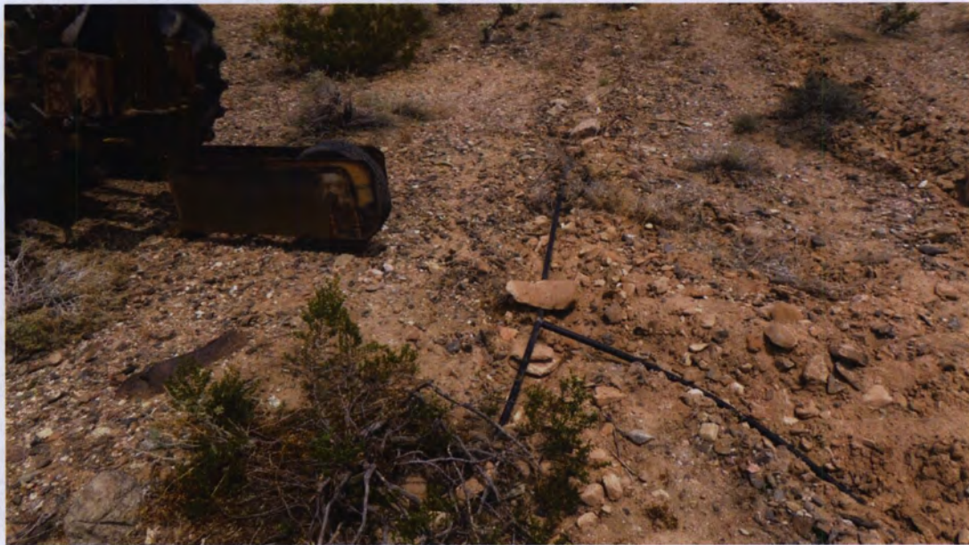
Image 11: Pipe tee at the tractor. The upper pipe (#1) heads northeast toward water source. The pipe to the right (#2) headed toward new water trough and pipe pointed straight down
