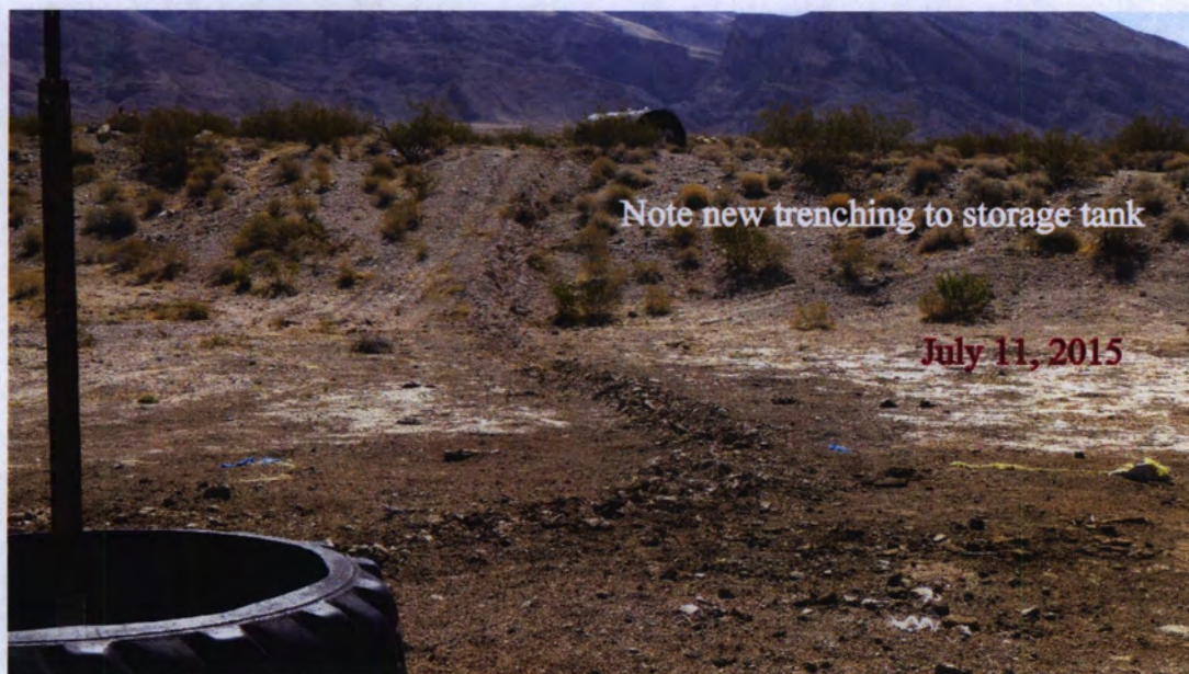
Image 18: Trenching to water tank. Photographed July 11, 2015.
