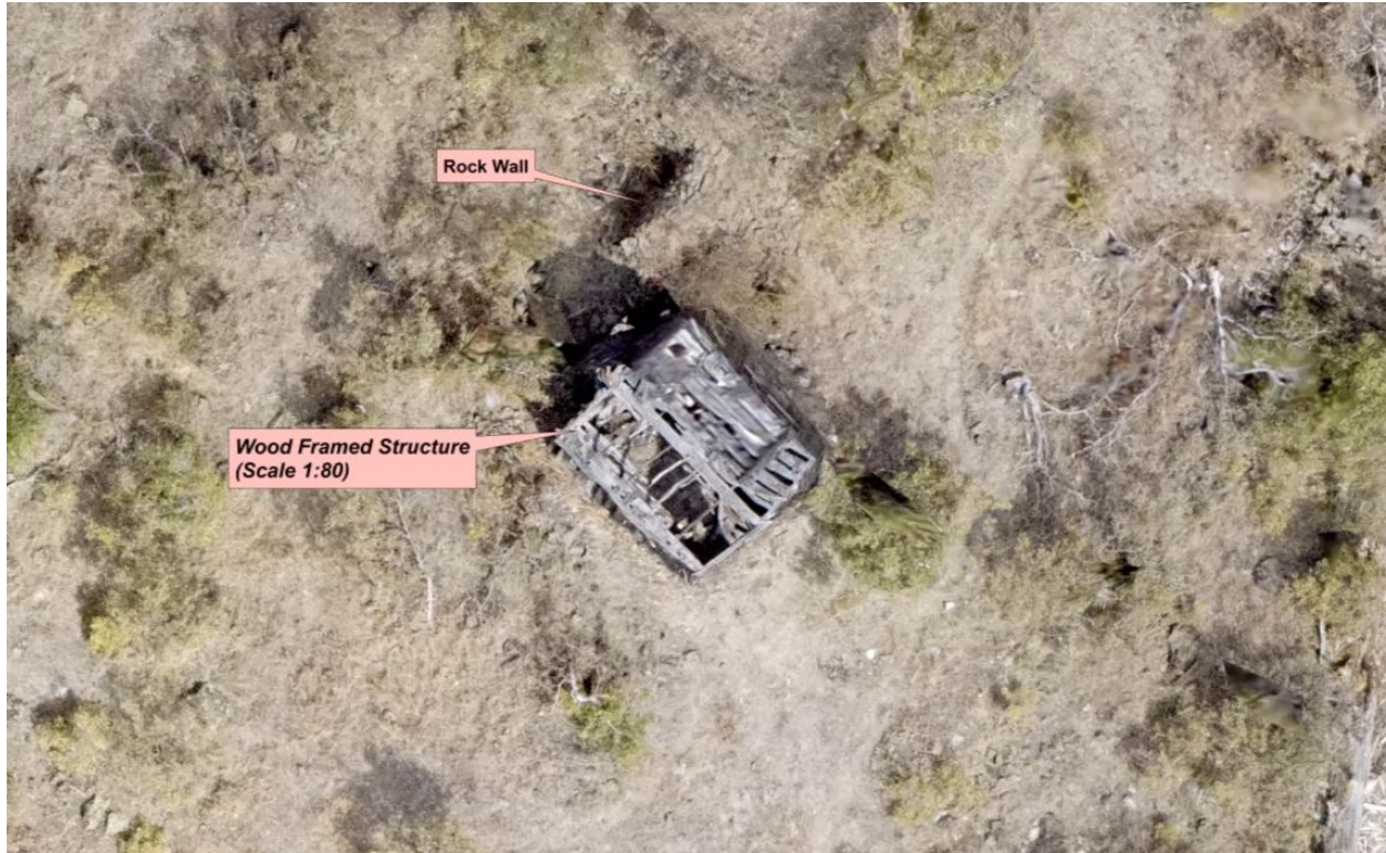
Photo 1: Historic Wood Frame Structure, Cottonwood Field Office
