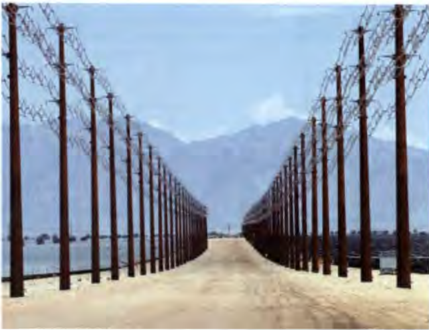
Transmission lines funnel energy from the Desert Sunlight solar farm to the Red Bluff substation near Desert Center, about an hour east of the Coachella Valley, on Aug. 20, 2014. (Photo: Crystal Chatham/The Desert Sun)
