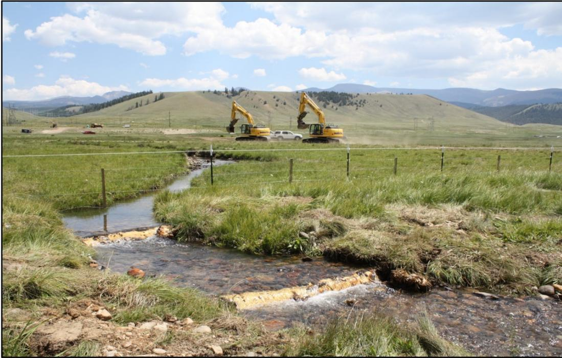
**Construction activities at the upper Arkansas River excavated pools, created stream riffles, and added woody debris and boulders to create improved feeding and spawning areas in the river. (FWS photo)**
