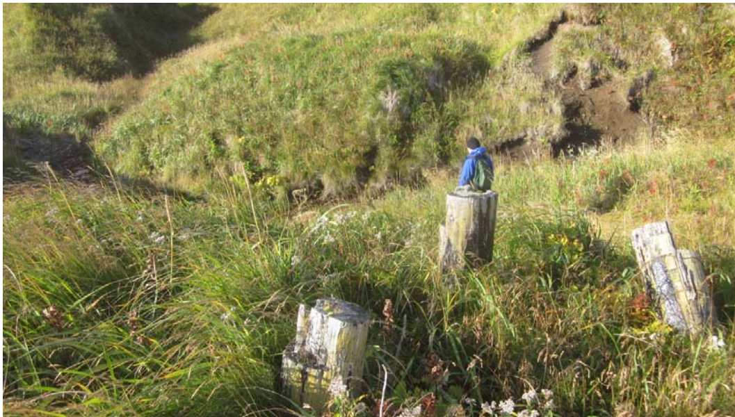
Figure 7: Upper Bank Pilings
