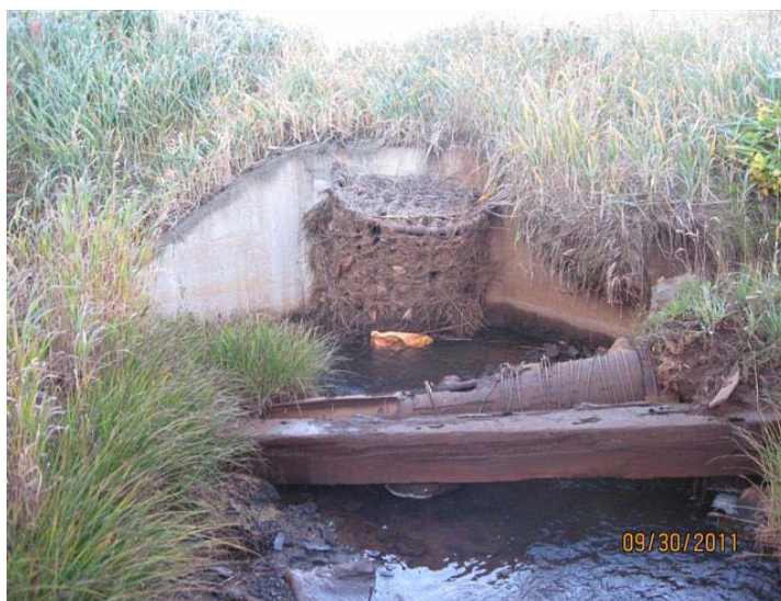
Figure 3: Wood stave pipe and timber
