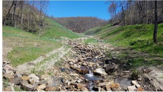
*Wolfden Run after reclamation showing the stabilized stream banks and reconstructed stream channel which employed geomorphic stream design techniques.*
