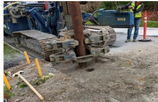
*Installation of grout pillars to create a bulkhead underground.*
