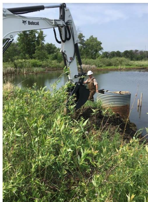
Active management of land and water resources supports conservation and wildlife dependent recreation. At Rice Lake NWR (MN), installation of a beaver deterrent helps maintain appropriate water levels and prevents flooding. Credit: USFWS
