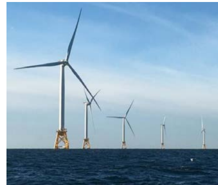
Block Island Wind Farm offshore Rhode Island
