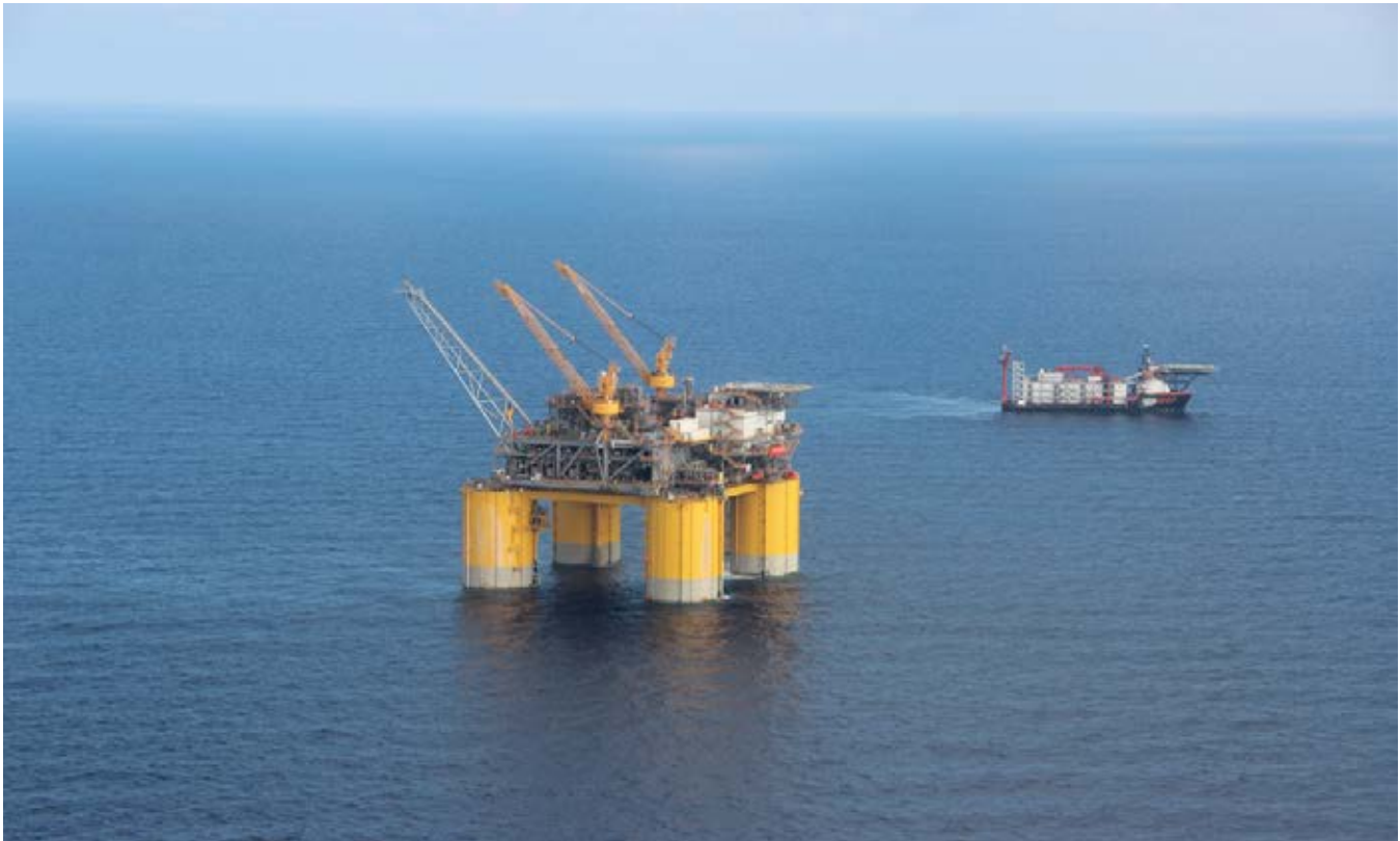
The Hess Stampede, located in the Gulf of Mexico, south of Houma, LA
