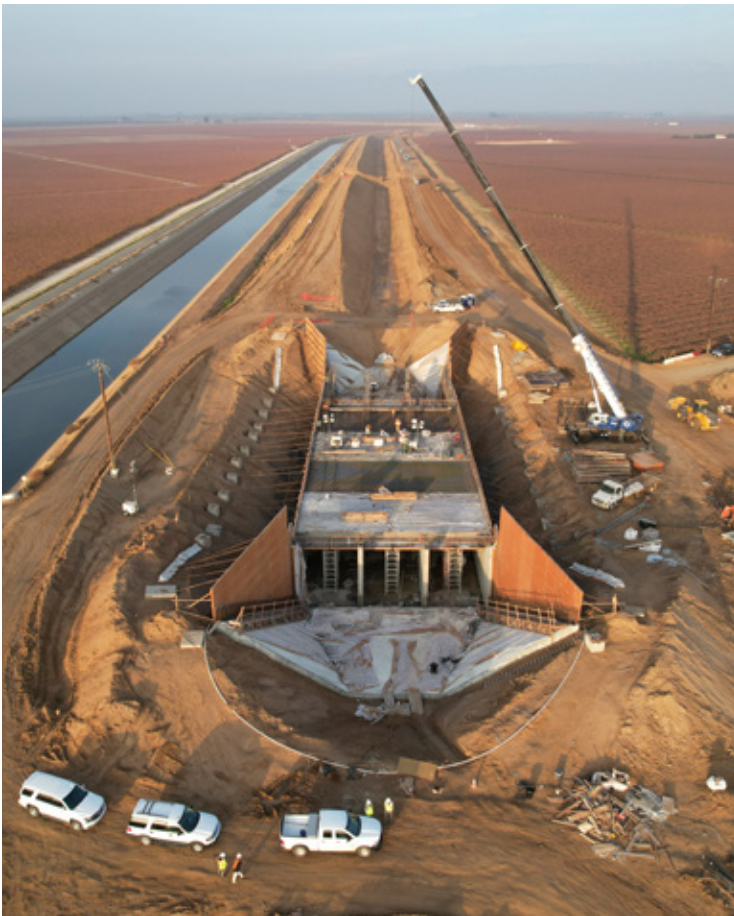
Construction at Friant-Kern Canal Phase 1 in Central California.
