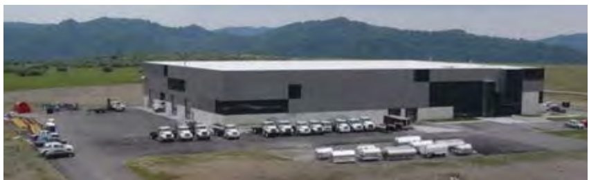
Marions Branch Industrial Park in Pike County, KY.
