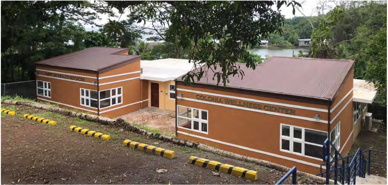
The new Colonia Wellness Center, which was completed in November 2021 and was jointly funded by OIA Compact Funds and the Government of Japan, in FSM. OIA Photo.
