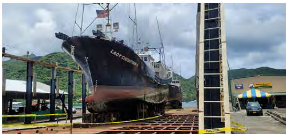
American Samoa Shipyard Authority 3000-ton slipway, which can now haul up to two boats. The last time this was possible was roughly 6 years ago.
