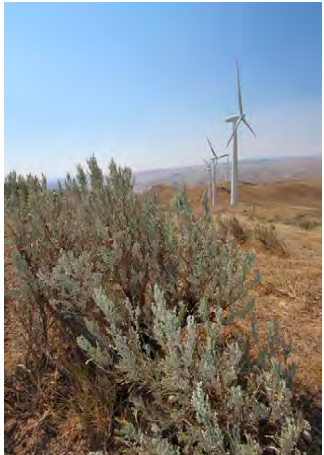
Lime Wind Energy Project in Oregon.
