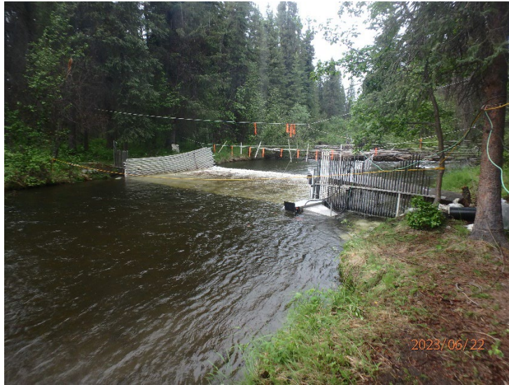
Tanada Creek Salmon Weir, 2023
