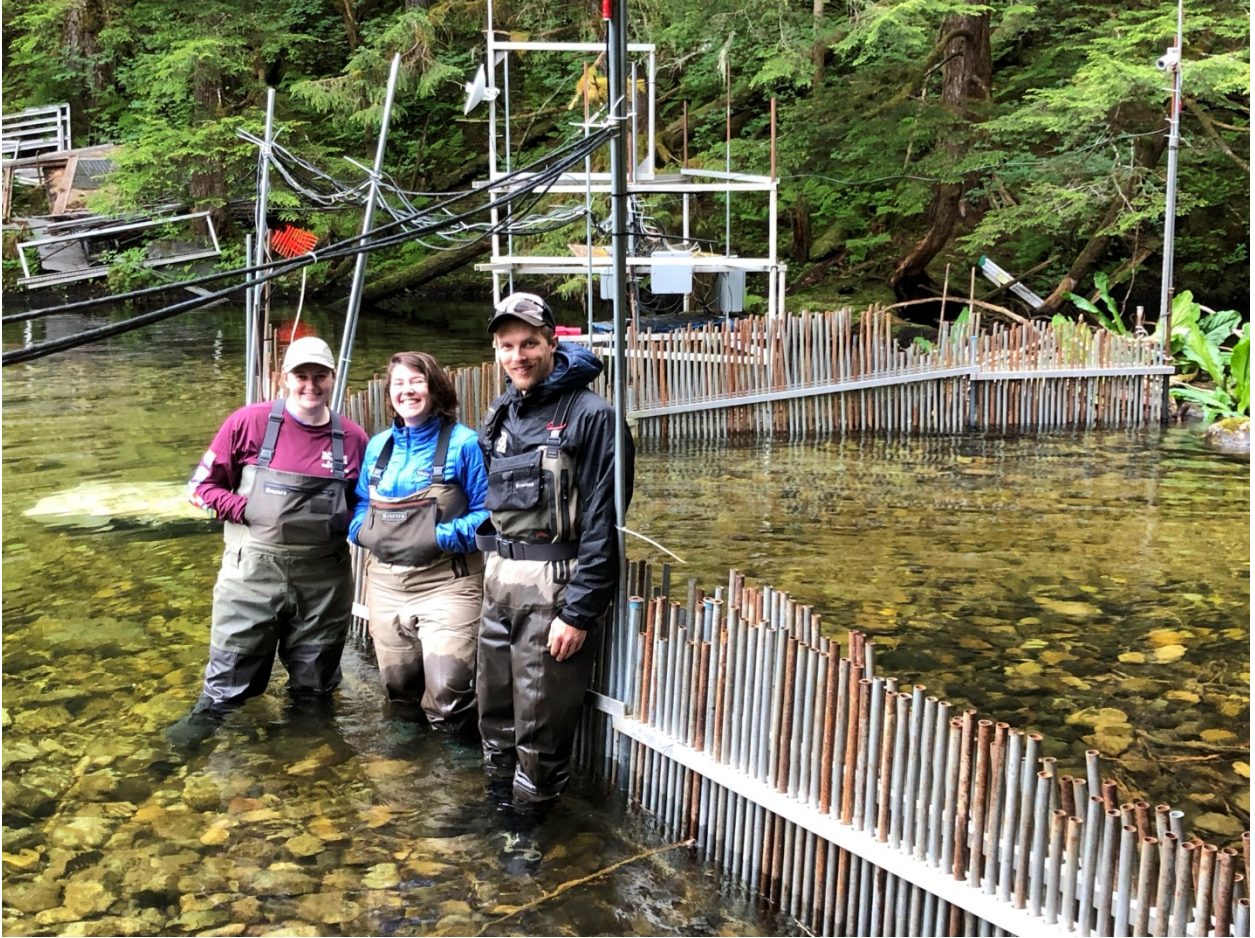
Figure 1. The Forest Service crew at the newly installed Neva Lake weir, June 29, 2021.
