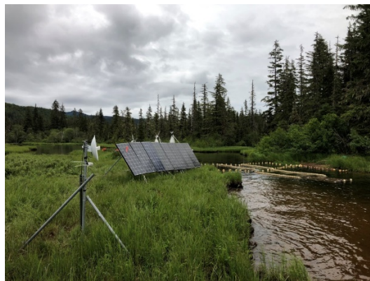
Figure 3. The video weir at the outlet of Sitkoh Lake, July 9, 2020.
