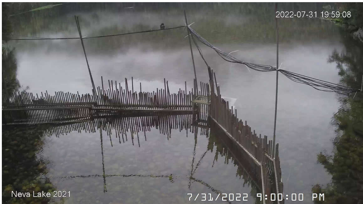
Figure 3. A foggy evening at the Neva Lake weir, July 31, 2022.
