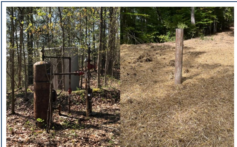
Figure 42. Mower Lumber #1 wellsite, Gauley River NRA, West Virginia – Before & After Plugging.
