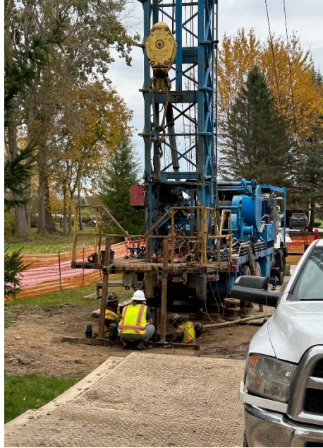
Contractors plugging the Burg J1 well in Alden, NY.
