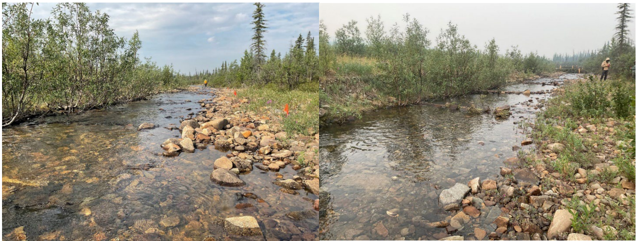
Figure 1. We experimented with post-less log structures to create step-pool features in a riffle dominated stream. These were quick and easy to create.
