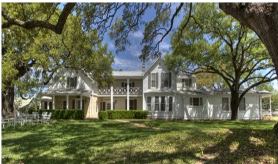
Texas White House. Photo credit: NPS
