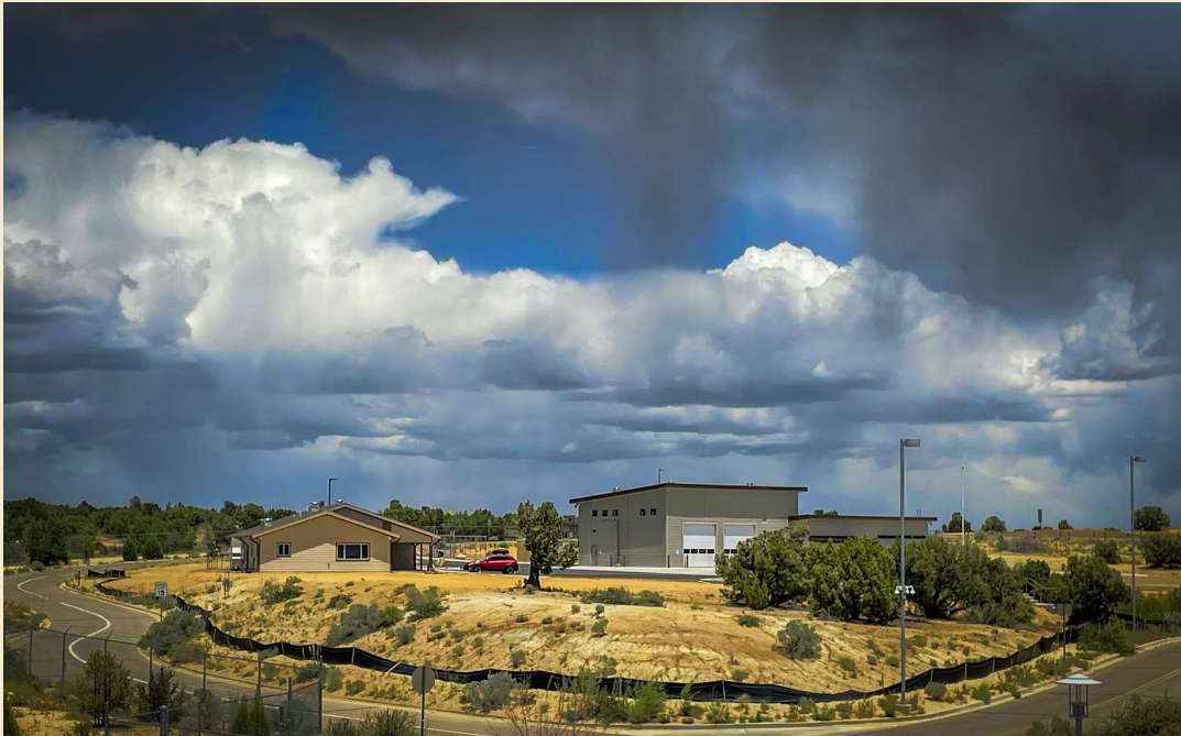
A new fire station and crew quarters constructed by BLM can be seen from the Farmington district office, New Mexico. (Photo by BLM.)
