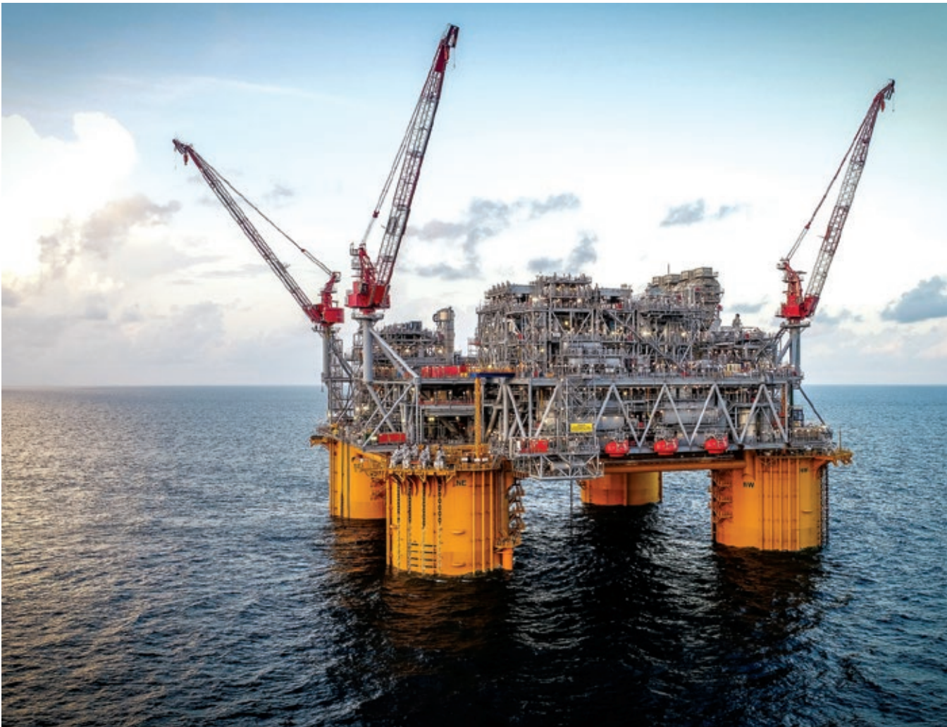
An oil and gas facility in the Gulf of Mexico.
