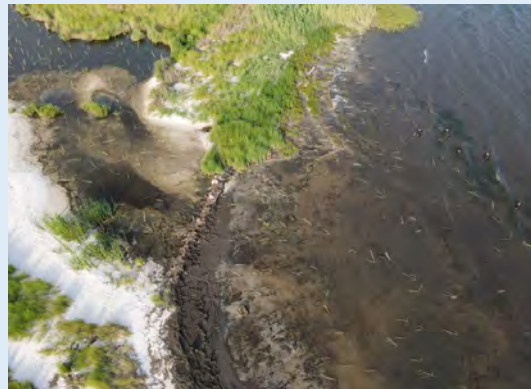
Bags of recycled glass in place, FWS photo
