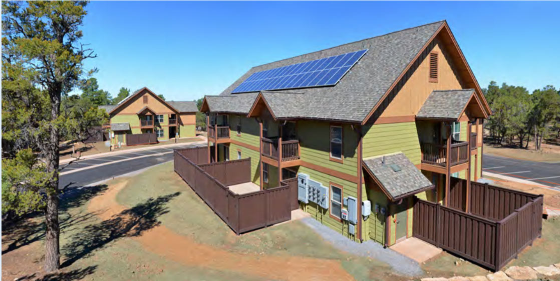
High-efficiency LEED Platinum-certified employee housing at Grand Canyon National Park. NPS/Michael Quinn
