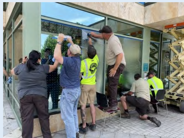
Employees installing prevention material at Patuxent Research Refuge, MD. FWS photo
