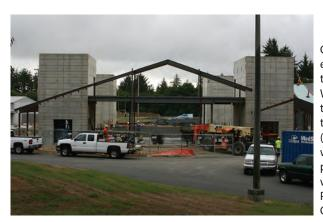
Construction of the first engineered tsunami refuge takes place in Westport, WA, in 2015. The completed tsunami refuge will span the flat roof of a gymnasium (9 meters above ground), with doors at ground level providing access to stairs within the corner towers. Photo credit: Sonya Miller, Ocosta School District
